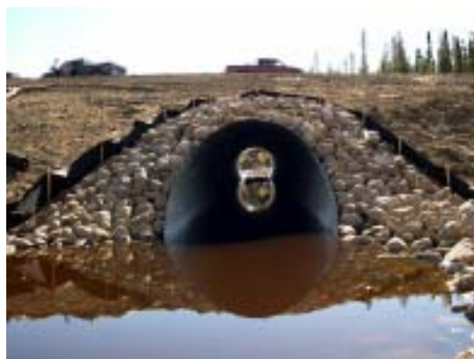
Figure 17. Outlet of culvert showing fillslope armouring and geotextile fencing.
