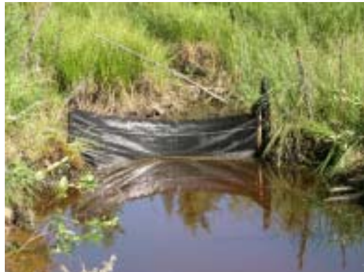
Figure 4. Fence made of geotextile near the outlet of diversion trench.
