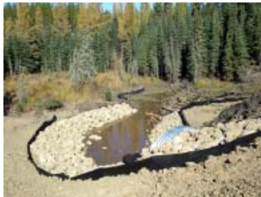
Figure 16. Outlet of culvert showing streambank armouring.
