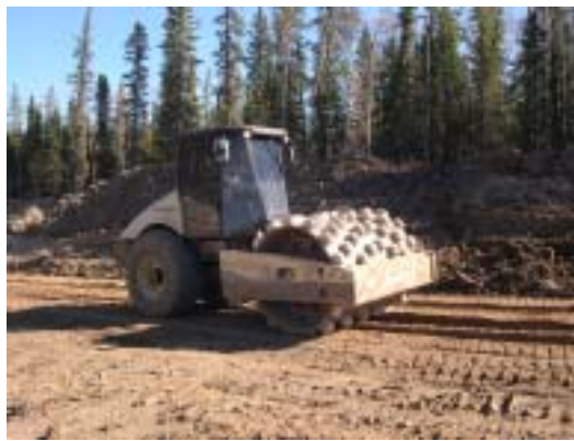
Figure 6. Vibrating-drum pad-foot roller used for compaction during various stages of construction.
