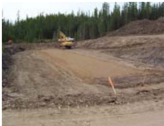
Figure 7. Sandy bedding prepared to a level surface (photo courtesy of Alberta-Pacific).
