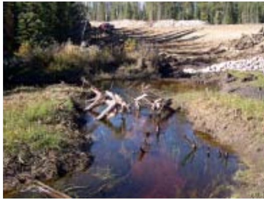
Figure 19. Root wads placed upstream of culvert within main channel of stream.
