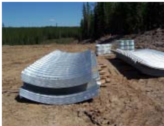
Figure 8. Unassembled culvert plates and buckets containing bolts (photo courtesy of Alberta-Pacific).
