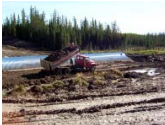
Figure 11. End-dump truck delivering backfill material (photo courtesy of Alberta-Pacific).
