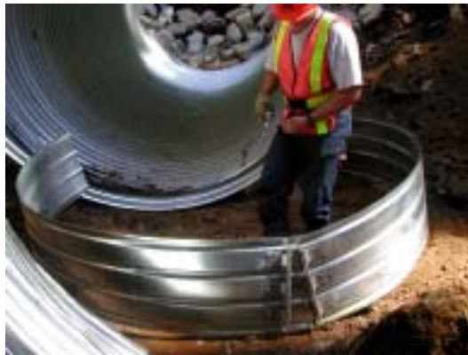
Figure 5. Two sections of the three-piece coupler being loosely joined together.
