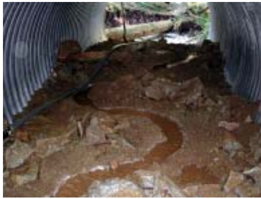
Figure 10. Final simulated streambed surface showing meandering low-flow channel between rock spurs.
