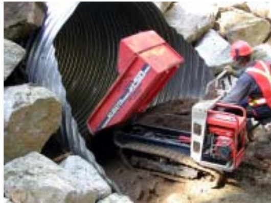
Figure 9. Wheelbarrow delivering infill material near the inlet of the culvert.
