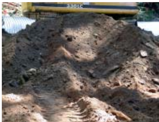
Figure 2. Material for bedding, backfill, and infill was predominantly coarse sand.
