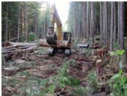
Figure 1. Excavator smoothing the surface of the corduroy trail.
