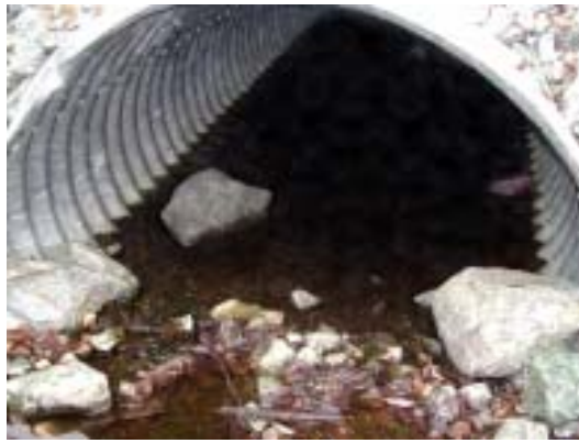
Figure 3b. Outlet of embedded culvert.
