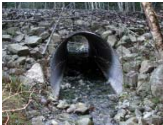
Figure 1b. Inlet of embedded culvert.
