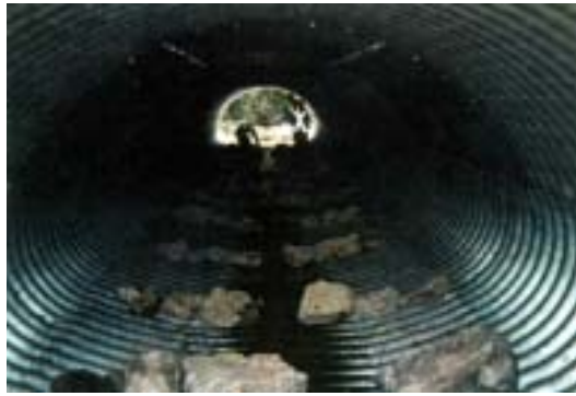
Figure 6b. Hand-placed boulders during installation (photo courtesy of Slocan Group, Mackenzie).
