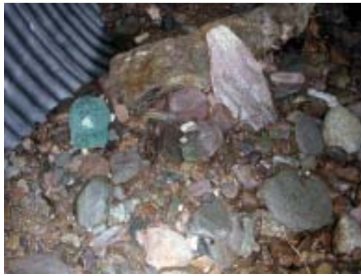
Figure 9b. Various sizes of aggregate within the culvert (hat can be used for scale).
