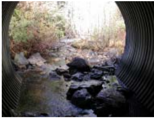
Figure 8b. Outlet of embedded culvert.
