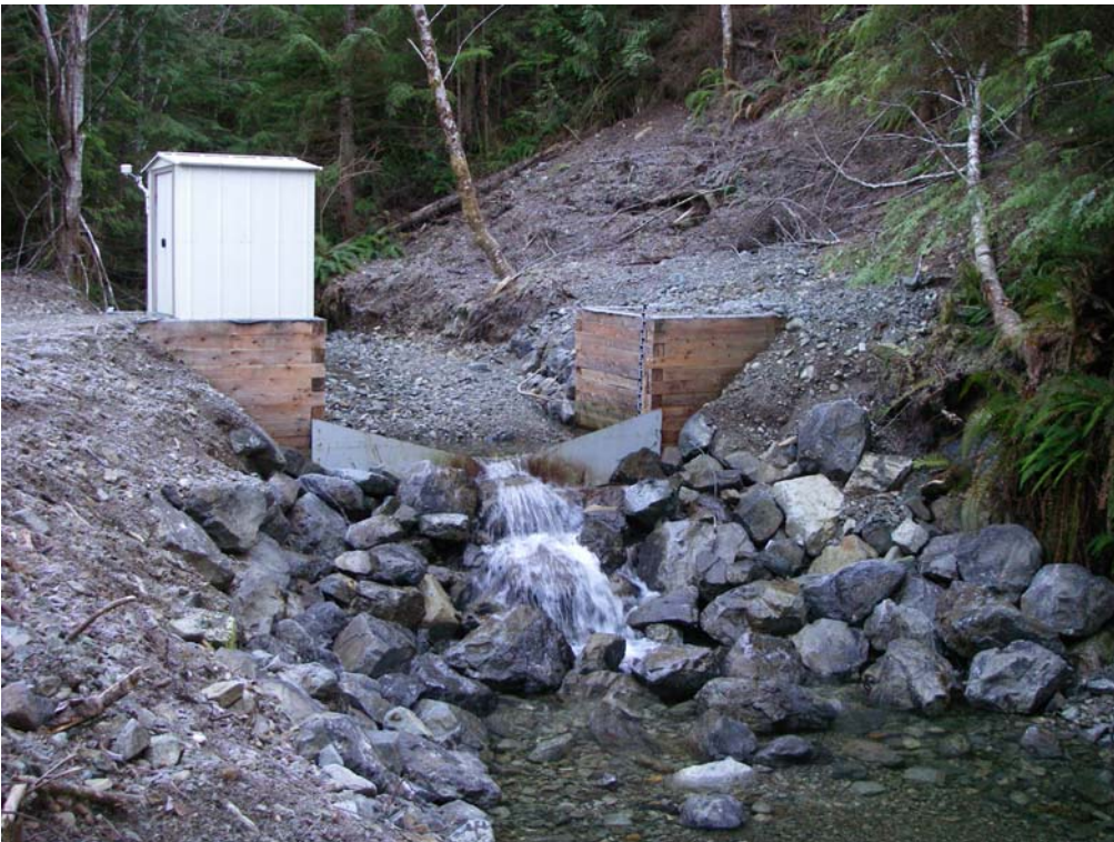
C Weir, control sub-basin, January 2008.
