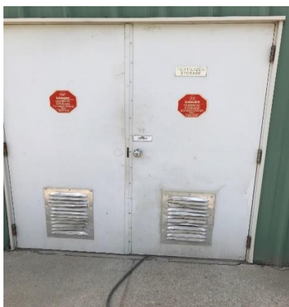
Figure 4a. and 4b. Example of a pesticide storage facility that was adequately locked, signed, and vented to the outside (left image). Example of a pesticide stored in manufacturer packaging with original label (right image).
