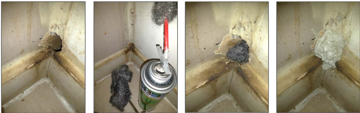
Figure 7. Example of exclusion work, an alternative to pesticides, for control of rodents performed by a technician
