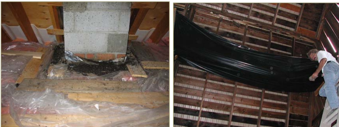
MODIFICATIONS FOR BAT ROOST SITES INCLUDING PLASTIC IN ATTIC TO FACILITATE GUANO REMOVAL AND REDUCE SMELL (TOP) AND A TARP TO PREVENT GUANO FROM FALLING HAY (BOTTOM).
