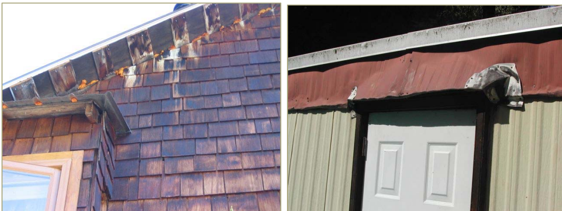
BAT ROOST UNDER SHAKES (LEFT) OR FLASHING (RIGHT). BATS MAY USE GAPS WITH SPACES LARGER THAN A FINGER WIDTH.
