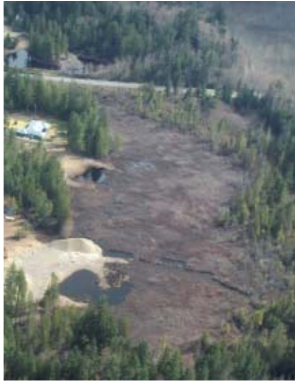
Plate 1: Polygon N1400 - Wetland in rural land use category Disturbed by cutting of vegetation, fill encroachment and excavation.
