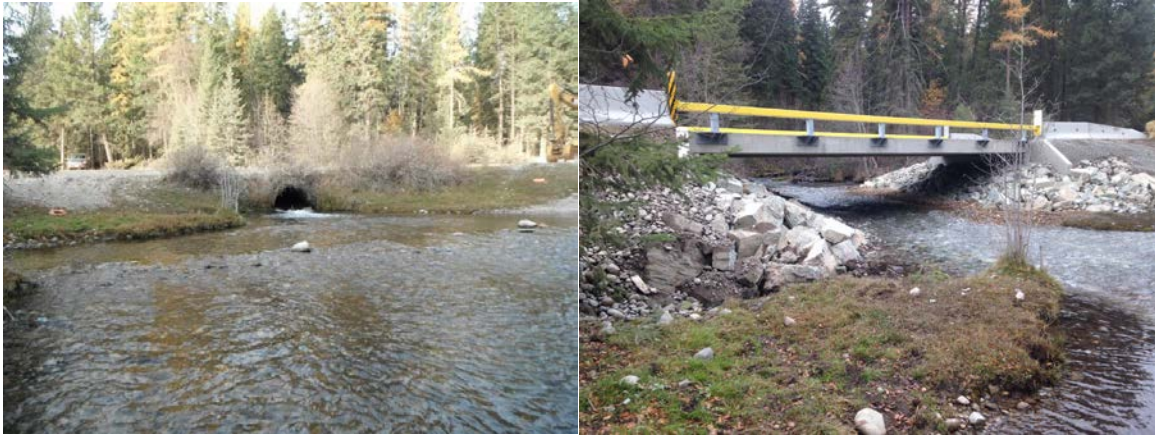
Photo: Plumbob Creek Crossing – before and after
