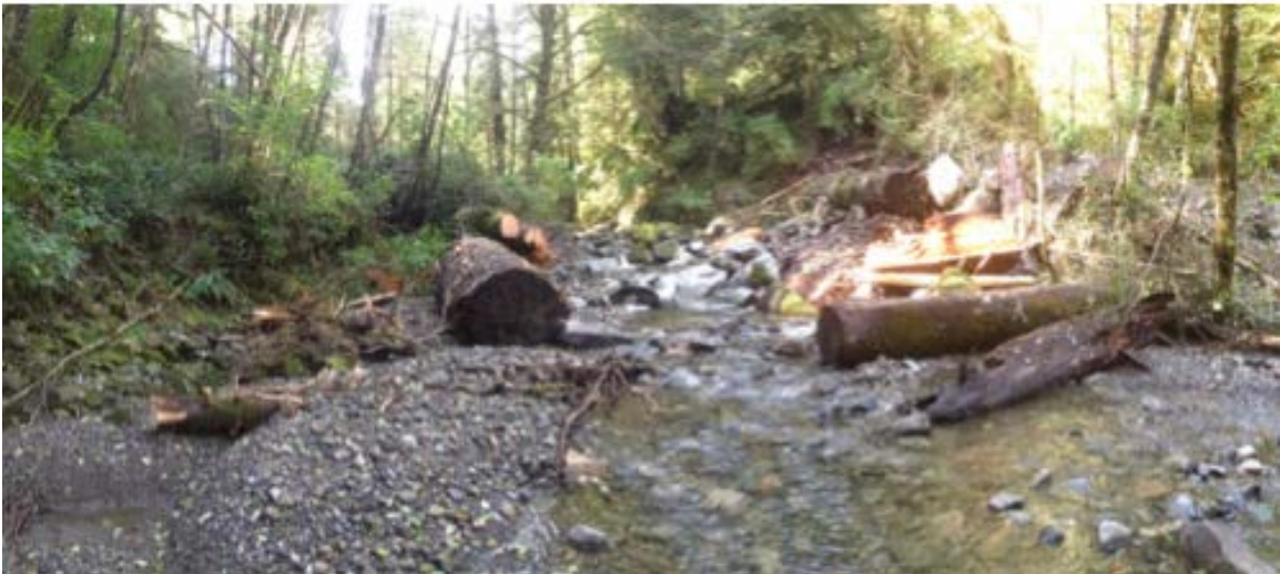
Upper photo: Clint Creek dam before the project Lower photo: Clint Creek dam removed due to the project
