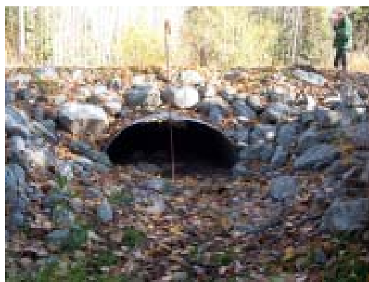
Figure 5c. Inlet of embedded culvert.
