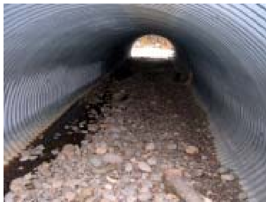
Figure 6b. Looking towards outlet of embedded culvert showing cobble-sized bedload.
