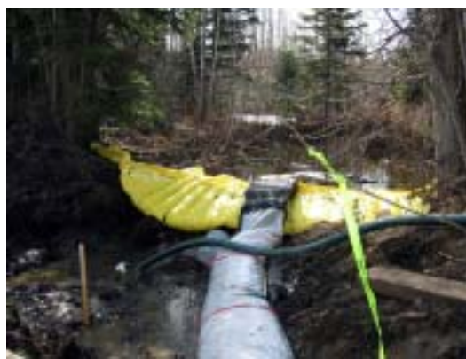
Figure 5b. Water-Gate™ dam with the overflow diverter tunnel (photo courtesy of BCMOF).
