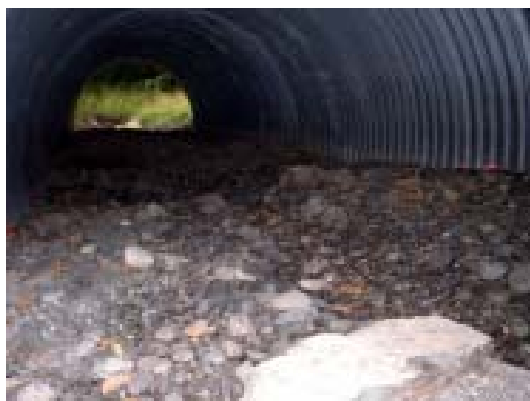
Figure 1a. Looking towards inlet of embedded culvert.
