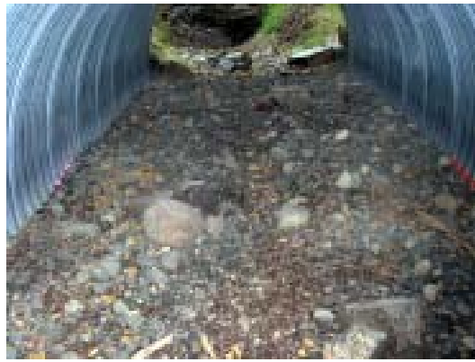
Figure 1b. Looking towards outlet of culvert.
