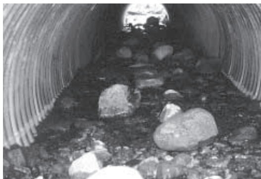
Figure 12. Final simulated streambed within the CSP, showing range of material sizes and streamflow spread across the width of the streambed.
