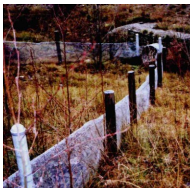
Design structures such as this 'toad tunnel' to allow amphibians safe passage under a highways. PHOTO: MARLENE CASKEY
