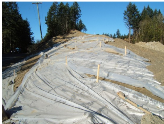
Prevent erosion and sedimentation. PHOTO: JUDITH CULLINGTON
