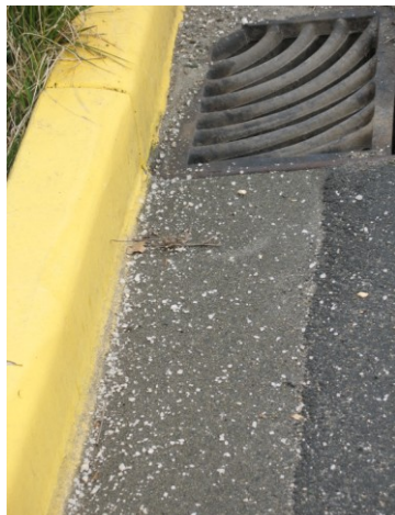
Use alternatives to road salt where runoff could impact wetland water quality. PHOTO: ROBERT COX
