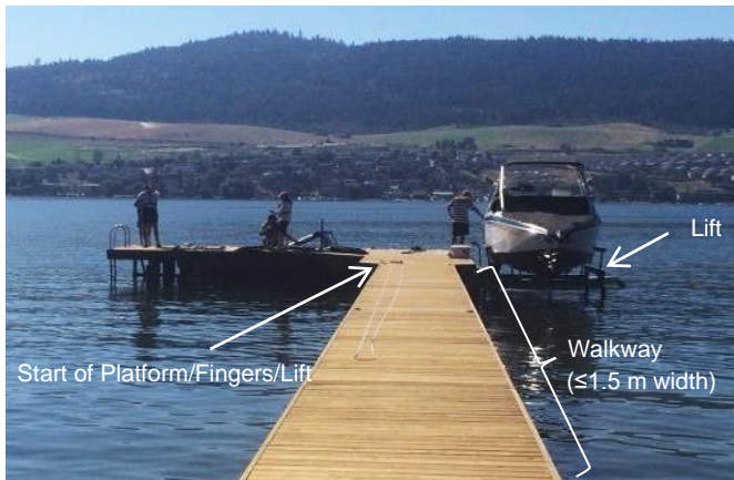
Example of Dock delineating Walkway, Platform and Lift
