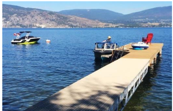
Dock in Red Zone constructed with Light Penetrating Decking
