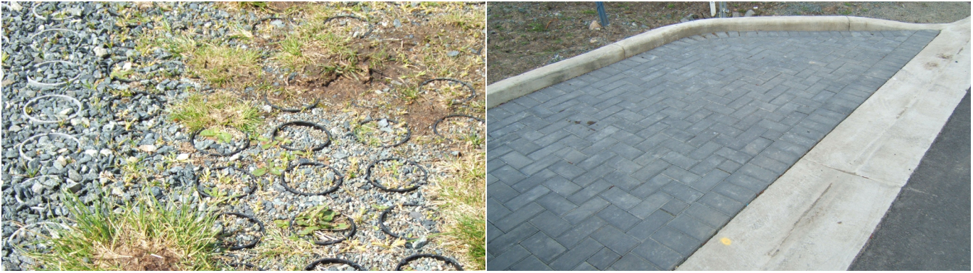
In high traffic areas, use permeable paving such as this gravel pave (left) or bricks (right)
