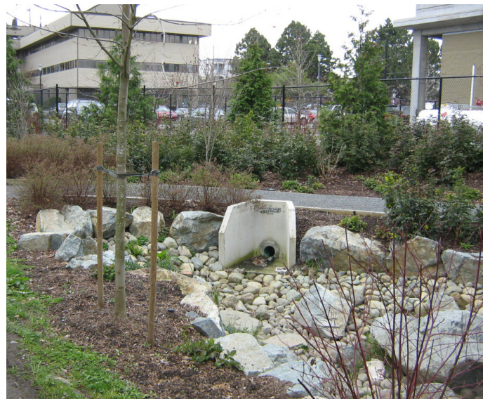
Construct raingardens to treat stormwater
