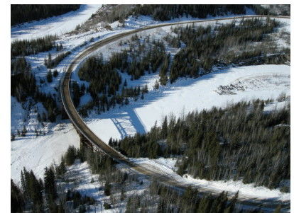
Kiskatinaw curved bridge. Photo: C. Thiessen.
