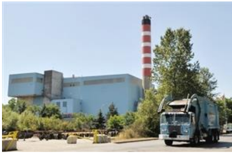
Fig. 4.1.9 Metro Vancouver’s South Incinerator Facility
