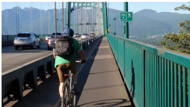
Lions Gate Bridge – Hwy 1A/99, Vancouver
