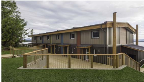
Bella Bella Staff Housing Complex (Vancouver Coastal Health)
