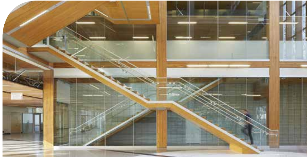
Image 4: The Earth Systems Sciences Building at the University of BC makes use of timber-concrete composite systems, with concrete topping contributing to the performance of the cross-laminated timber floor panels and supporting glulam beams. The feature stair (above) cantilevers into the atrium, with glued-in HSK plates connecting CLT elements. For more information, refer to case study by naturally:wood 14 (Image courtesy of Martin Tessler).
