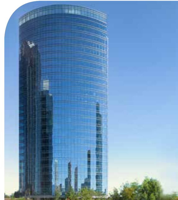
Image 7: Portland-limestone cement was used in the construction of the LEED Platinum Metrotower III in Burnaby, B.C. (Image courtesy of © Ledcor. All rights reserved).
