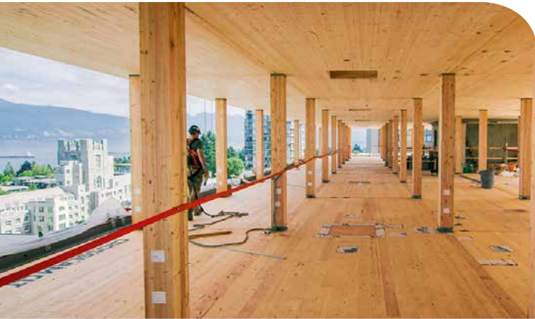
Image 2: UBC currently boasts the tallest modern hybrid wood building in the world - Brock Commons Tallwood, which features 17-storeys of timber structure over a single concrete level. See case study in Appendix A. Please also refer to case study by naturally:wood 11 (Image courtesy of www.naturallywood.com ).
