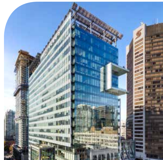
Image 8: Portland-limestone cement was used in the construction of Telus Garden, a 22-storey office building in downtown Vancouver. The dramatic entrance features a sweeping roof with curved glulam beams (Image courtesy of Henriquez Partner Architects).
