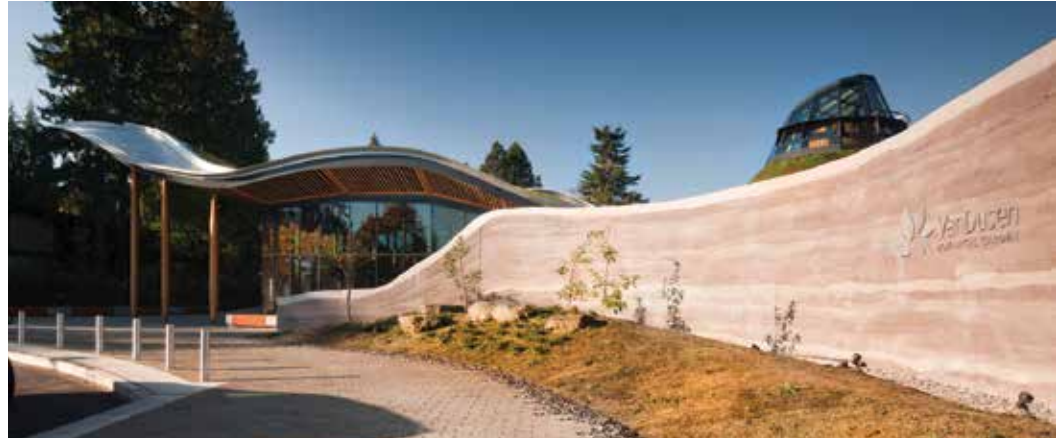
The VanDusen Botanical Garden Visitor Centre uses low-carbon building materials such as wood and stabilized rammed earth (Image Courtesy of Sirewall 49 ).
