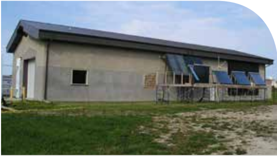
Straw bale Research Building, University of Manitoba, Winnipeg, Manitoba. (Image courtesy of University of Manitoba).
