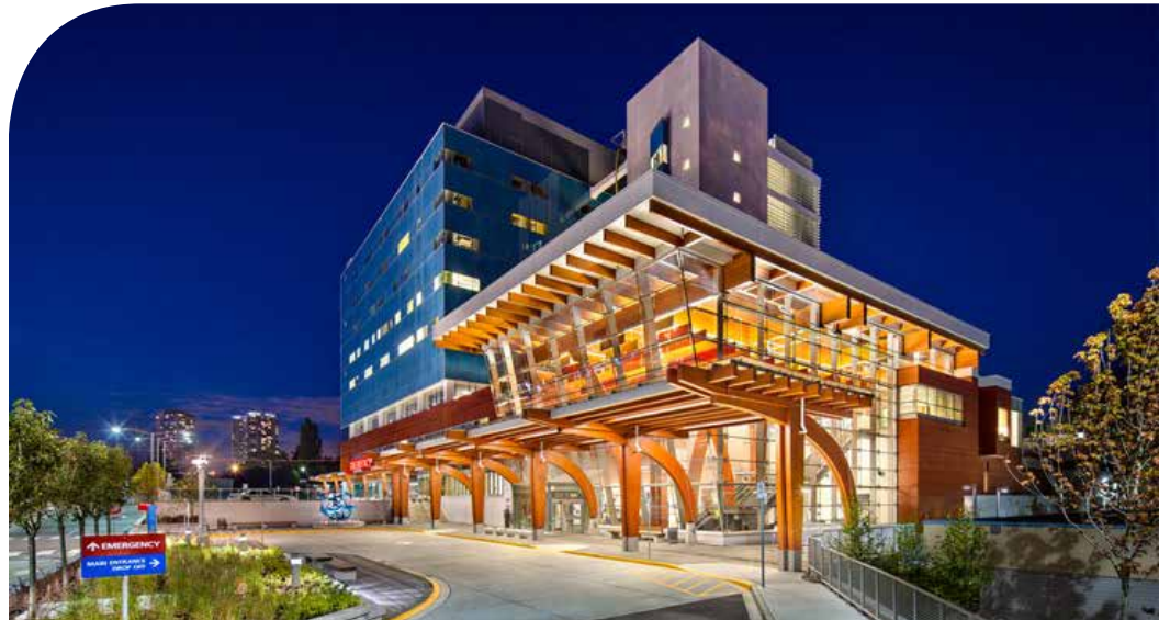
Image: Surrey Memorial Critical Care Tower incorporate many wood elements into the design 83 (Image courtesy of EllisDon).
