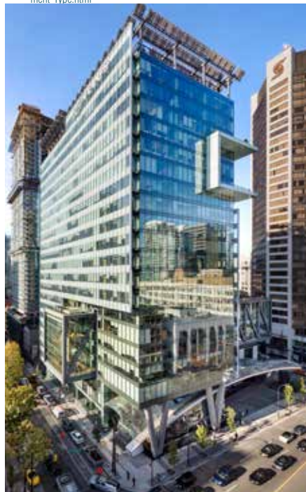
Portland-limestone cement was used in the construction of TELUS Garden in Vancouver. The dramatic entrance features a sweeping roof with curved glulam beams (Image courtesy of Henriquez Partners Architects).
