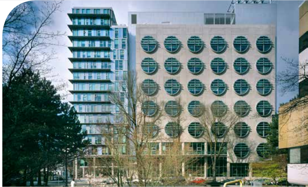
The B.C. Cancer Research Centre in Vancouver was one of the first LEED Canada certified projects, achieving LEED Gold certification in 2005. (Image courtesy of IBI Group/Henriquez Partners Architects in Joint Venture. Photographer: Nic Lehoux).
