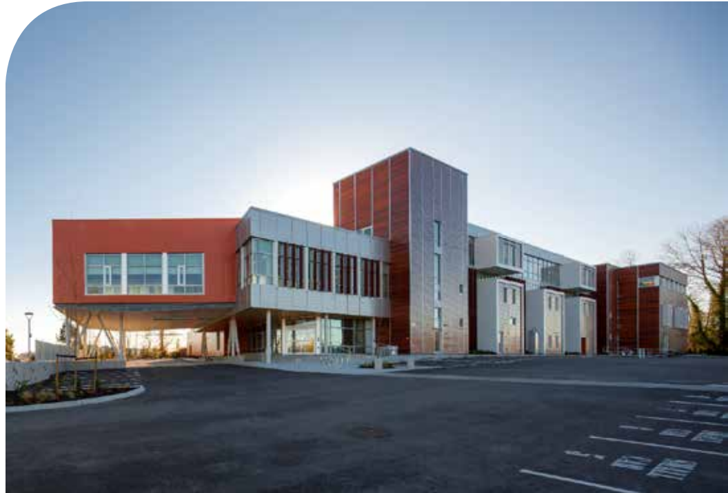
The Pacific Autism Family Centre in Richmond, B.C., used pre-fabricated NLT floor panels supported on a glulam post-and-beam structure and NLT elevator shafts. (Image courtesy of naturally:wood).
