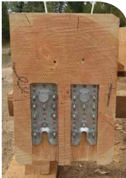
Example of a pre-engineered aluminum dovetail connector during installation. (Image courtesy of My-Ti-Con).
