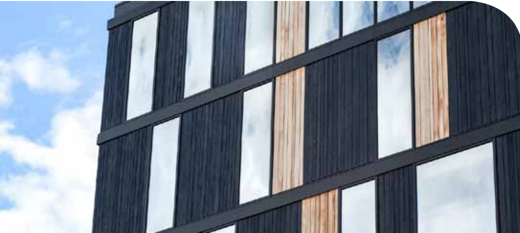
The Wood Innovation Design Centre at the University of Northern British Columbia in downtown Prince George used the Shou Sugi Ban technique of creating a charred wood finish (Image courtesy of Ed White).
