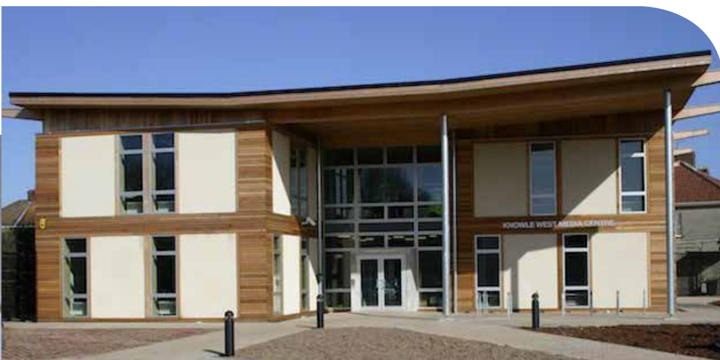
Knowle West Media Centre, Bristol, UK, using ModCell prefabricated straw bale panels (Image courtesy of ModCell).
