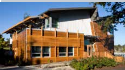
Operations Centre, Gulf Islands National Park Reserve, Sidney, B.C. was the first project to be awarded LEED Platinum in B.C. (2006) (Image courtesy of McFarland Marceau Architects Ltd. and Willie Perez, P. Eng.).
