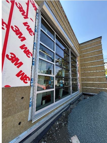
SARDIS SECONDARY NEW ADDITON BUILDING ENVELOPE DETAILS
