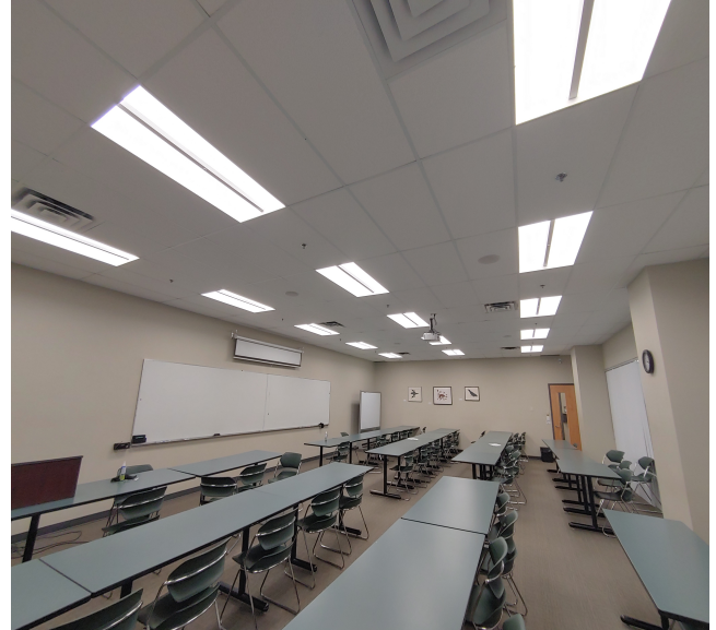
Figure 1: New Classroom Fixtures
