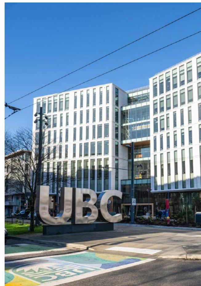
Gateway Health Building
