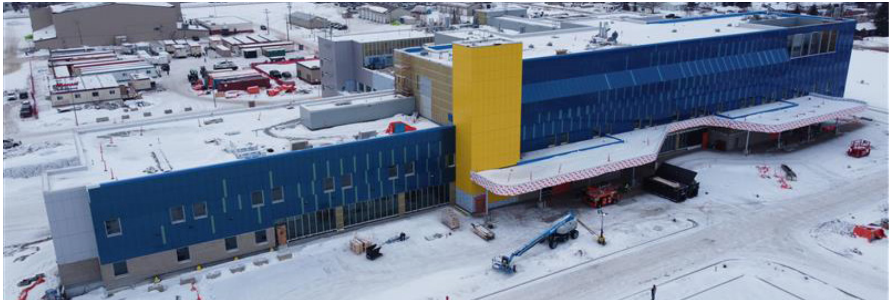
The new Dawson Creek Hospital, in development
