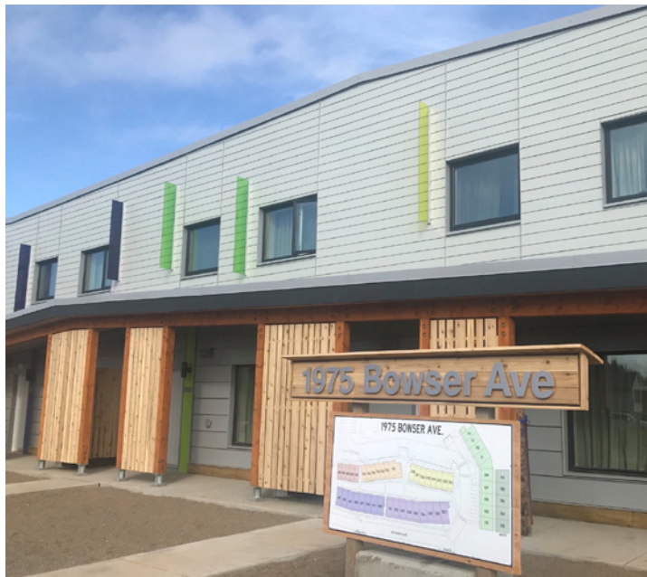
1975 Bowser Ave: Affordable, supportive housing managed by the Aboriginal Housing Society of Prince George.
