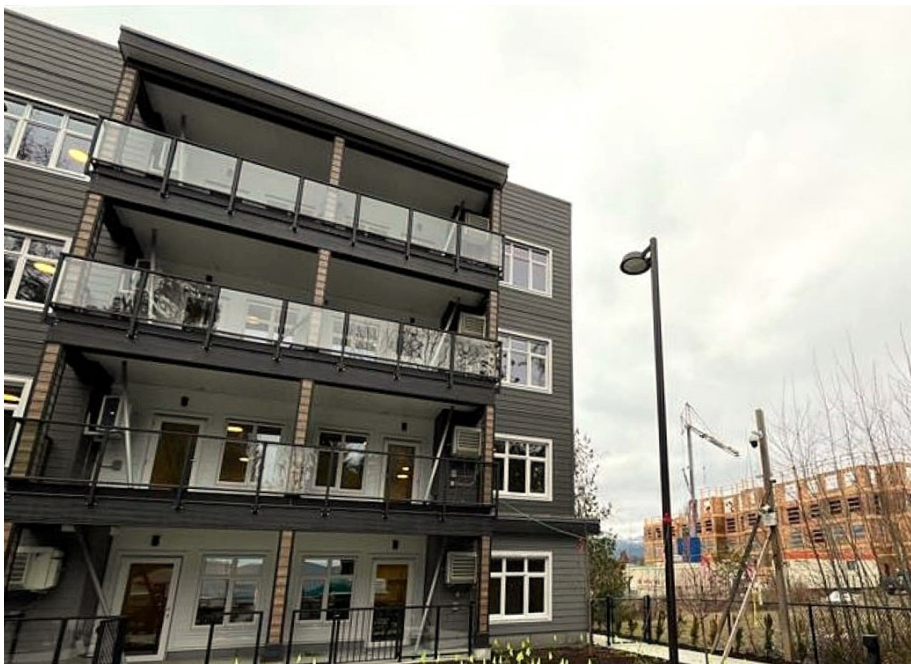
Eagle Valley Senior Housing: A BC Energy Step Code Step 3, fully electrified seniors' housing project featuring a high-performance building envelope to reduce energy demand and support low-carbon operation.
