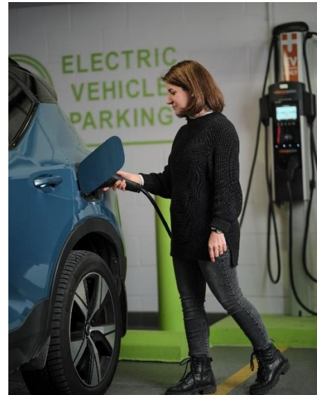
Electric vehicle (EV) charging station at the LDB Head Office.
