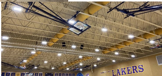
Lighting upgrade in gym
