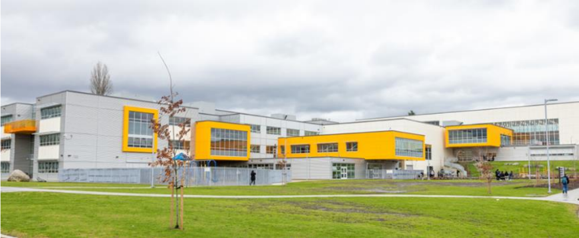
Figure 2: Burnaby North Secondary School- New Facility
