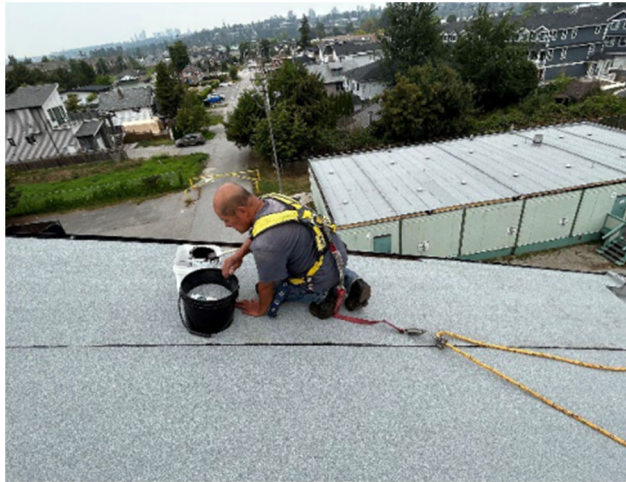
Finishing up the new roof at Queensborough Middle School
