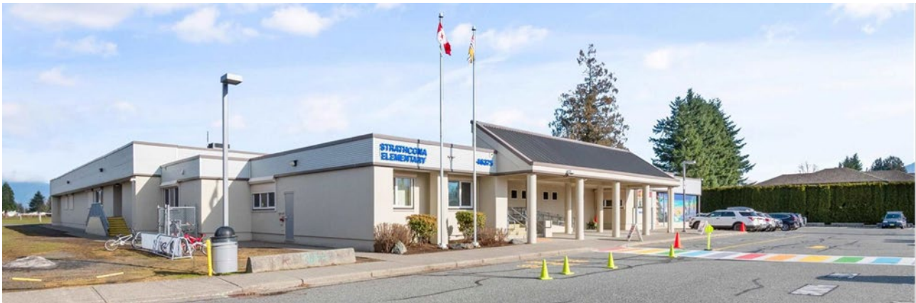
(Picture: above: Strathcona Elementary School, below: Strathcona Elementary Roof Top units)
