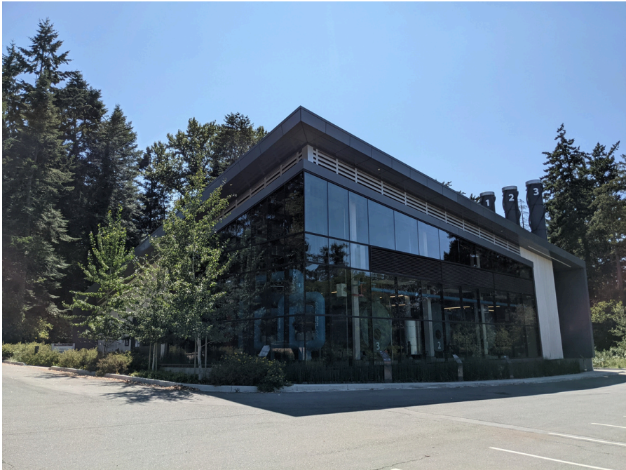
Image 1. The District Energy Plant completed construction in 2018 provides domestic hot water and space heating to 80% of the gross floor area across campus.
