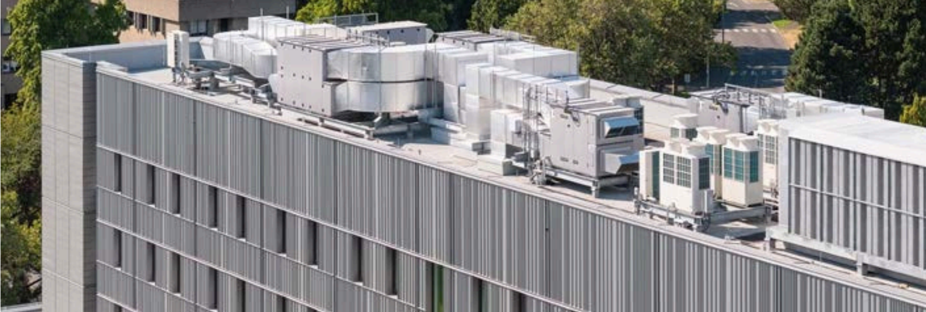
Image 3. The two new student housing buildings include solar shading features to prepare buildings for 2030 temperatures.
