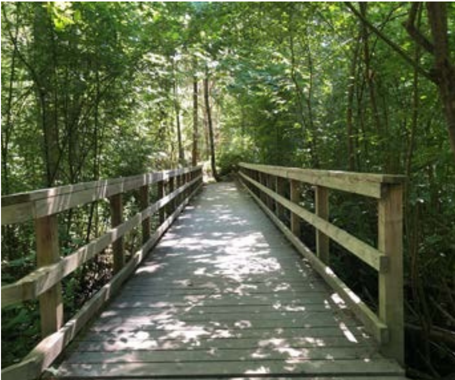
Image 6. Wooden bridge located in Bowker Creek Headwaters.
