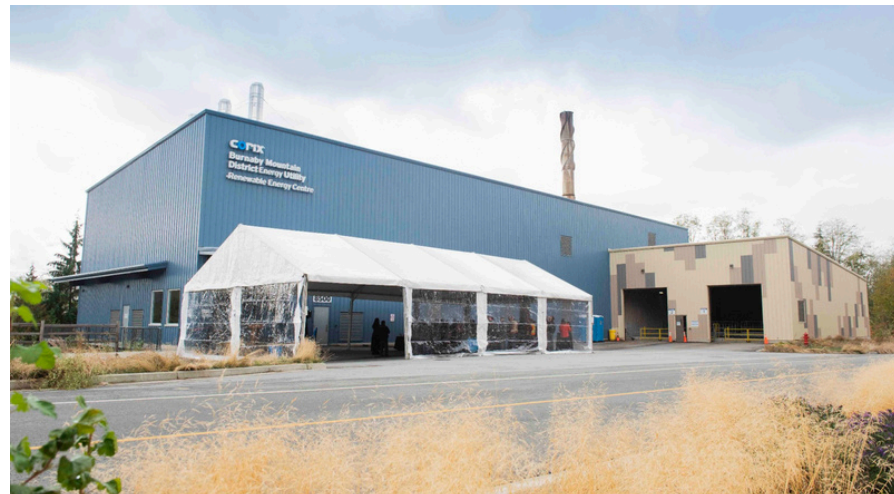
Figure 4 - SFU's Corix biomass plant on Burnaby campus.
