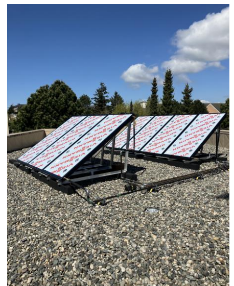
Photo 2: Peace Arch Hospital Solar thermal panel in preparation
