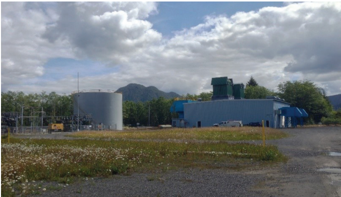
Prince Rupert Thermal Generating Station
