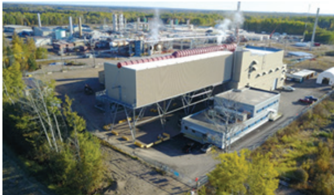
Fort Nelson Thermal Generating Station
