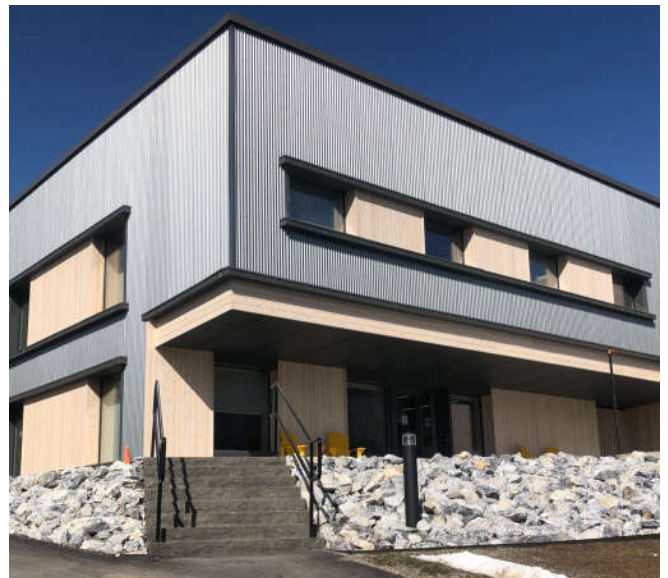
Figure 1: Facilities Management Building
