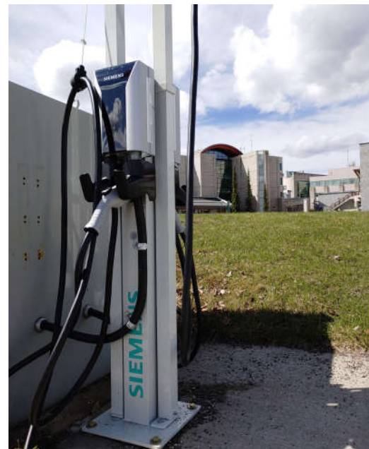
Figure 3: Level 2 Electric Vehicle Chargers
