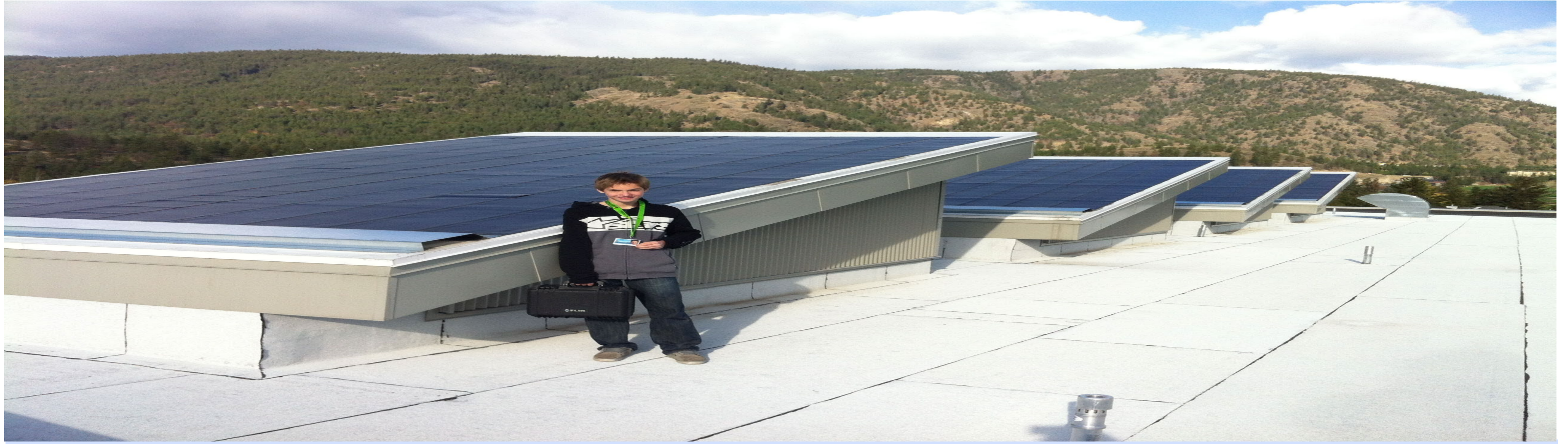
Shannon Lake Elementary School - 6 kWatt Solar Panel Installation - 60,000kWhrs of power saved of ten years of operation.
