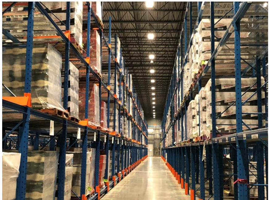
Liquor Warehouse, Delta, B.C.
