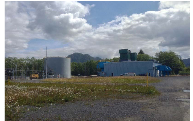
Prince Rupert Thermal Generating Station
