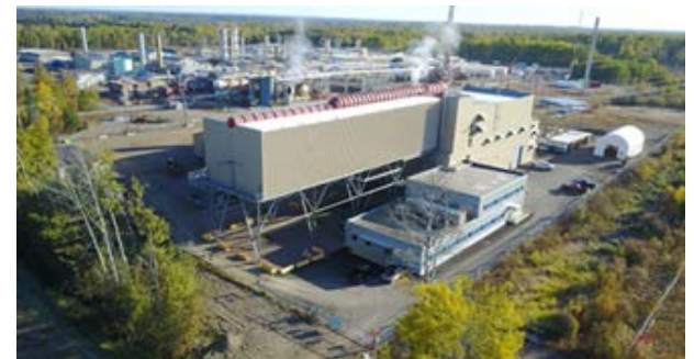
Fort Nelson Thermal Generating Station
