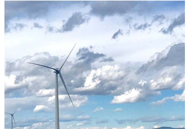
The 15 MW Zonnebeke Wind Project reached commercial operations in March 2021, and was developed as a partnership between West Moberly First Nations and Natural Forces. Photo by Natural Forces.
