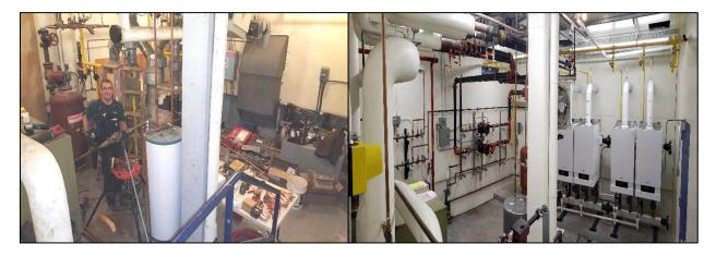
At Kitimat City High School (Cormorant School) the boiler plant and pump systems were replaced by inhouse staff. The new boilers are much more efficient and dependable to provide heat throughout the building. New direct-digital controls and recommissioning of the program for the HVAC system also contributes to a lower carbon footprint.
