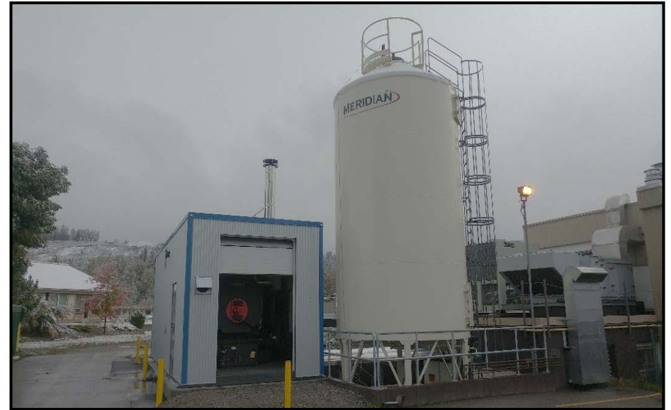
Containerized Biomass Boiler
