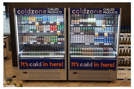
Open-front coolers at BCLS are equipped with a shade that is drawn at closing time every evening to reduce excessive cooling.
