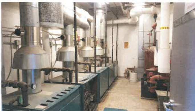
Old atmospheric boilers vs new condensing versions
