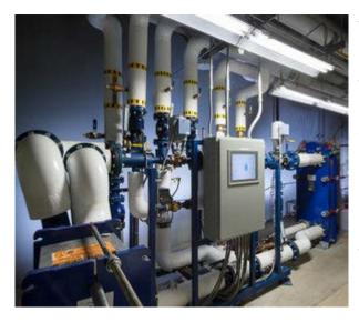
The design and construction took advantage of several state of the art technologies. A key feature being the physical location which allowed the Campus to connect to the City of Vancouver's Neighborhood Energy Utility System. The this "waste to energy" utility provides hot water for both Campus Heating and Domestic Water and eliminates the need for the University to burn fossil fuel for heating. Other features include:
