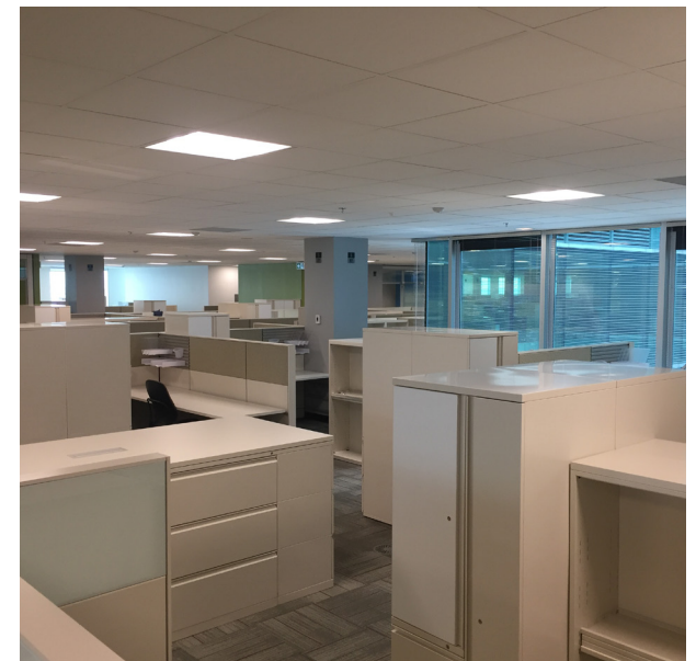
Office renovation at Edmonds campus.
