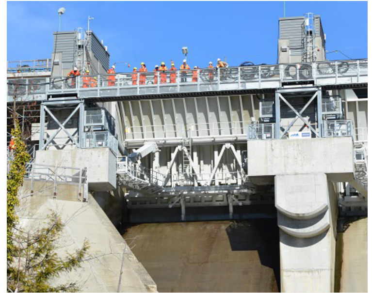
Last of the Ruskin Dam Spillways placed into service.
