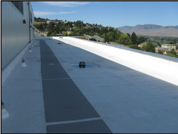
Example of reflective roof at Royal Inland Hospital, Kamloops, B.C.
