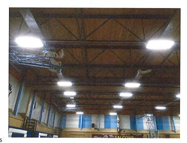
to 25w T-8s, vacancy sensors and from T-8 32w gymnasium lighting to dimmable LED fixtures. Exterior lighting upgrades included all new LED fixtures and dark campus programing.
