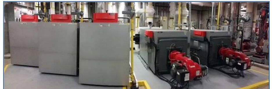
Powell River General Hospital: High Efficiency Boiler Upgrade.
