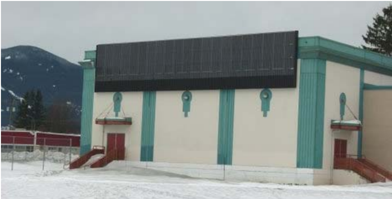
Solar Wall at Agassiz Elementary-Secondary School, Agassiz, BC
