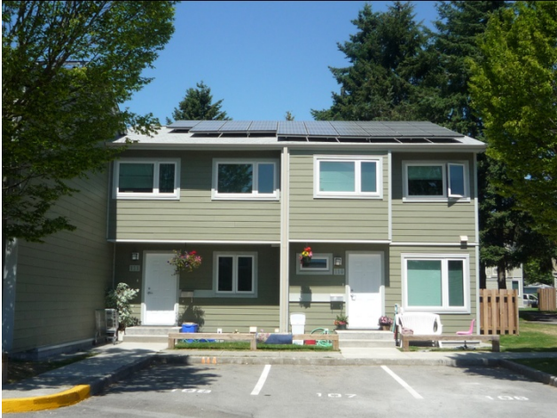
Roof top solar panels at Greenbrook
