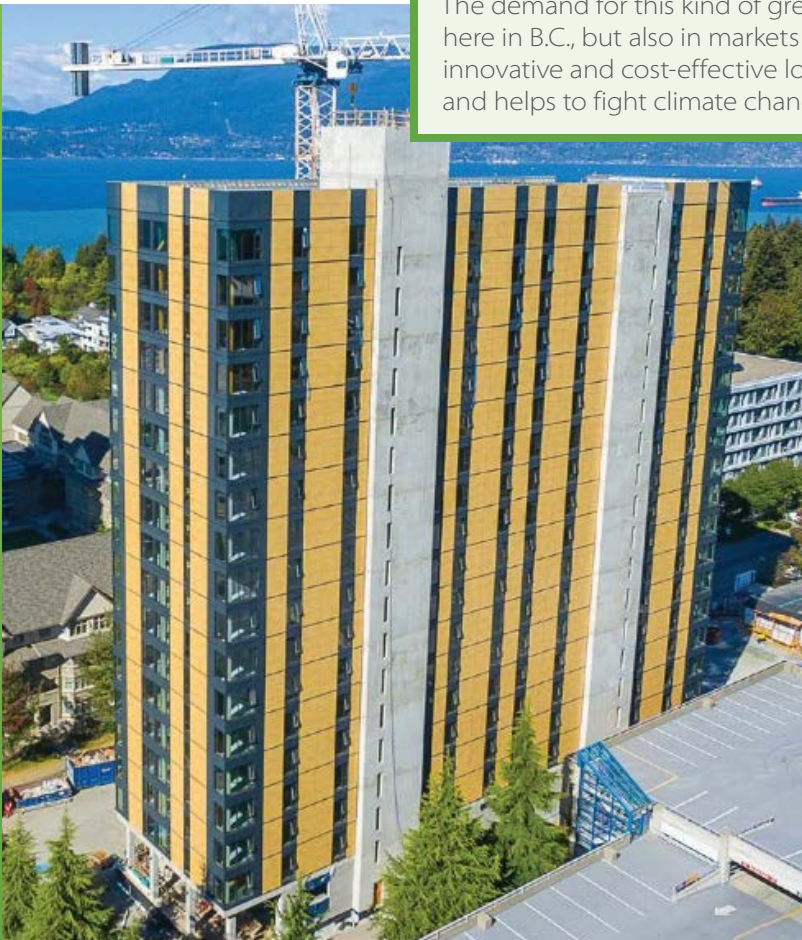
UBC's Brock Commons was built using mass timber supplied by Structurlam Mass Timber Corporation, and when completed in 2017, was the tallest wood building in the world, storing about 1060 tonnes of carbon.
